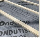
For guaranteed waterproofing, **ONDUTISS** is the preferred membrane of choice to install with the full range of Onduline's bituminous corrugated roof sheets.
