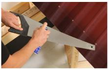
**Cutting with hand saw**Use a course bladed handsaw to cut
