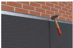
**3** FONDALINE® can be nailed directly to concrete only on levels where there is no risk of infiltration of damp or ground water.
