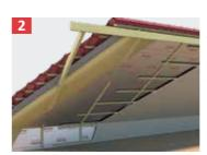
Fix ONDUTISS® BARRIER REFLEX vapour proof membrane to the roof with staples. Avoid any damage of the foil. Use ONDUTISS® double sided tape to seal hermetically all joints and all connections appropriately. According to your roofing system, fix ONDUTISS® BARRIER REFLEX bands in place by applying the supporting structure of the interior paneling, or by nailing counter battens above the membrane through to the rafters to protect the fixing area.
