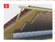
Roll out ONDUTISS® BARRIER REFLEX vapour proof membrane across the rafters, at the warm side of construction. Start from the bottom, always the printed side facing you. The overlap is indicated by lines or logo print.
