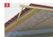
Fix ONDUTISS® BARRIER vapour proof membrane to the roof with staples. Avoid any damage of the foil. Use ONDUTISS® both double sided tape to seal hermetically all joints and all connections. According to your roofing system, fix ONDUTISS® BARRIER bands in place by applying the supporting structure of the interior paneling, or by nailing counter battens from above to the rafters to protect the fixing area.
