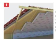
Roll out ONDUTISS® BARRIER vapour proof membrane across the rafters, at the warm side of construction. Start from the bottom, always the printed side facing you. The overlap is indicated by lines or logo print.
