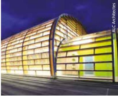
ONDUCLAIR® PC sheets are made of polycarbonate resin (thermoplastic resin).
